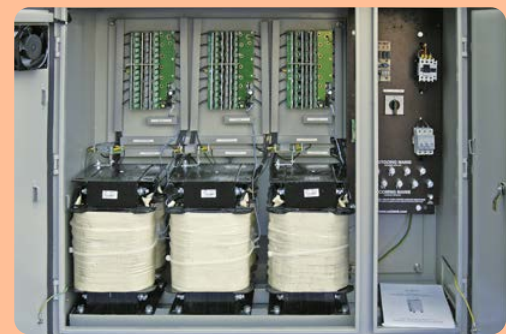
Internal components of an outdoor AVR
