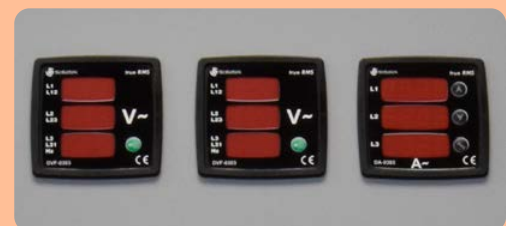
Internal AVR display panel with input, output and current digital displays
